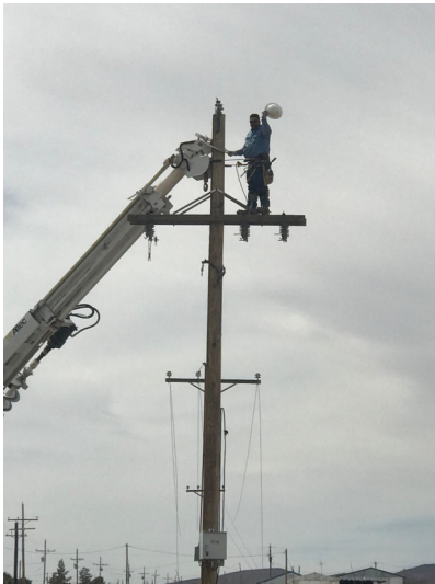
Journeyman lineman Cruz Villa
